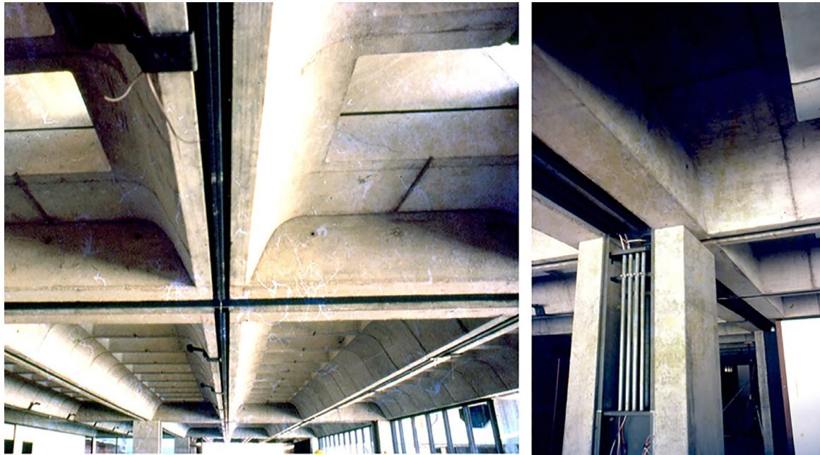
**Illustration 5 and 6.** Sarah/DF – ribbed slabs with ducts for wiring; double beams and columns for the passage of diverse installations.
