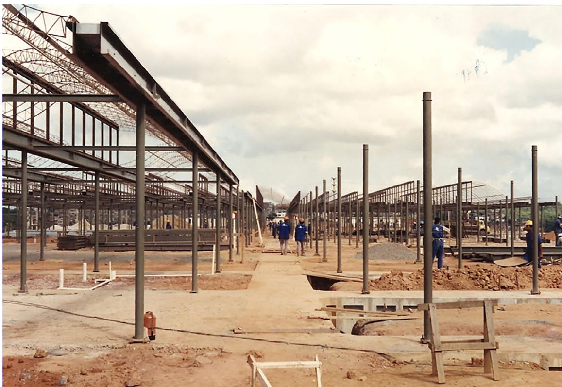
**Illustration 13.** Sarah/BA - assembly of double longitudinal beams and transversal tie beams.
