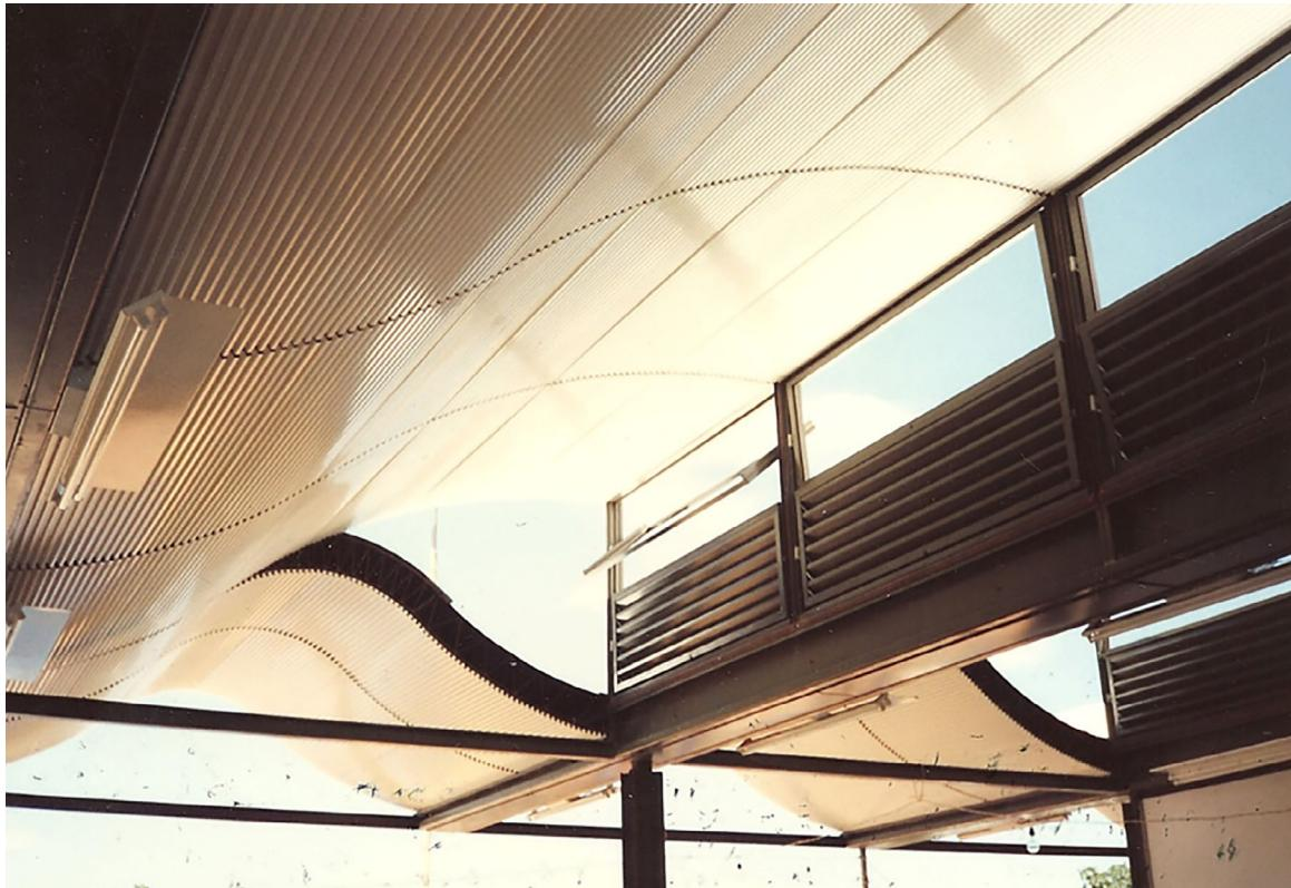
**Illustration 15.** Sarah/BA - double beams with attached light fixtures, tie beams and roof being assembled: foreground with shed; background, without shed (for balconies and air-conditioned rooms).
